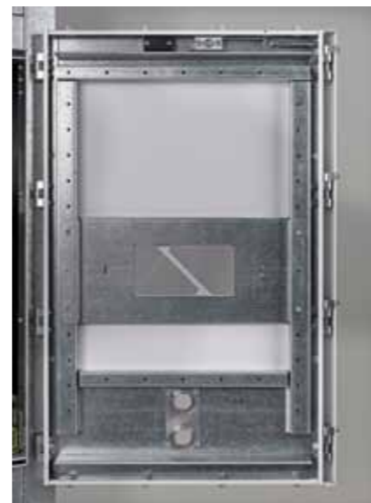
Properly designed labyrinths as well as additional steel sheets provide maximum operator safety in case of internal arc fault
